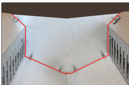
STEP 10: Apply caulking as shown on both ends and install.
