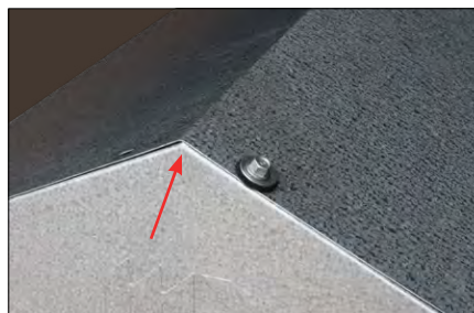
STEP 8: Slide end cap into place, making sure pre-punched holes and top break align. Using (1) screw, attach the end cap to hold into proper position. Repeat on opposite end of vent.
