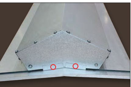
STEP 11: When installing, place end of vent on provided end skirt and center with peak. Fasten* to end cap and repeat on opposite end.
